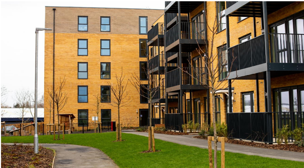
Errol Court, completed March 2021
